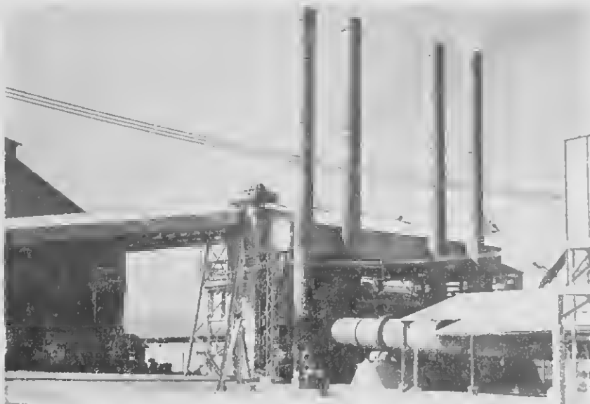
AT PARANAM is the second of the company's two major plants. The long circular machinery is the rotating drying kiln; metal grade bauxite passes through this.
